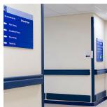
Wall protection systems are used to protect surfaces from damage caused by the general flow of pedestrian or wheeled traffic.
